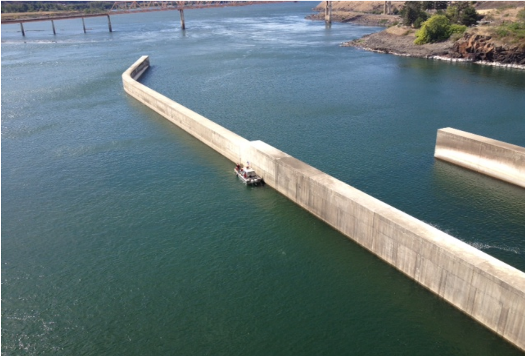
Dive inspection of spillwall to check for erosion.
